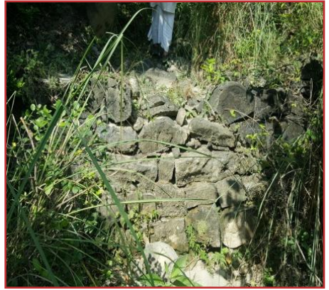
The check dam found in sector 22 of Lohgarh Fort
