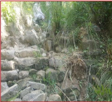
The check dam found in sector 18 of Lohgarh Fort.
