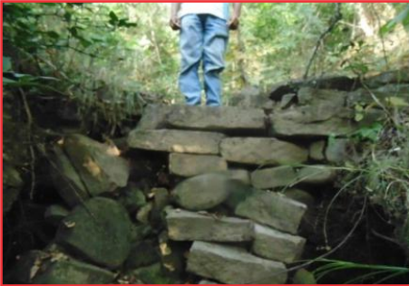
The check dam found in sector 5 of Lohgarh Fort.
