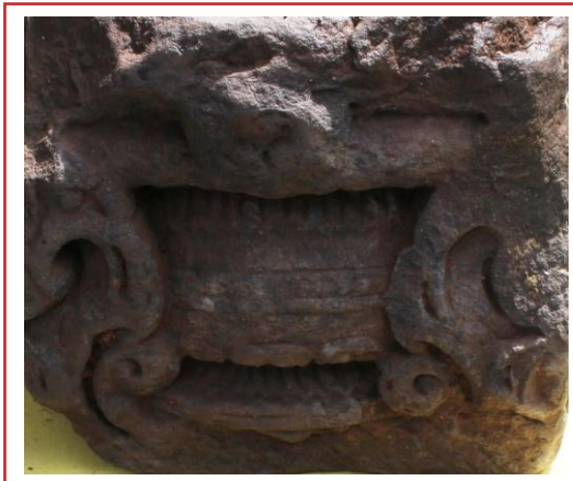
Dressed stone used for construction of fort Lohgarh. There is hole in every stone so that lime mortar can get its strength and each stone are bound with other one strongly.
