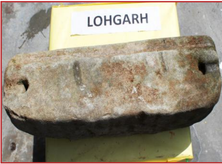
Dressed stone used for construction of fort Lohgarh. There is hole in every stone so that lime mortar can get its strength and each stone are bound with other one strongly.
