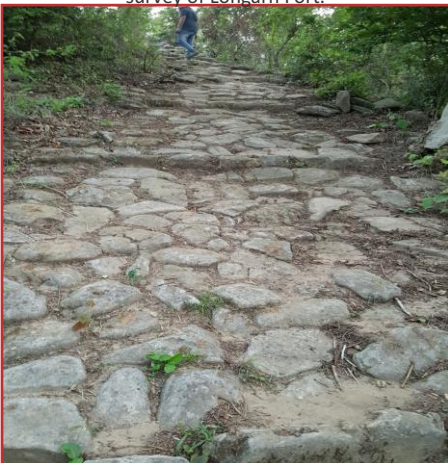
Ramp found in sector C-20
