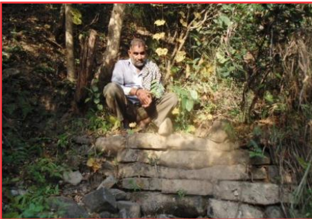
The check dam found in sector 6 of Lohgarh Fort.
