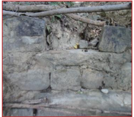
The check dam found in sector 23 of Lohgarh Fort.
