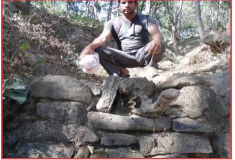
The check dam found in Sector 4 of Lohgarh Fort.
