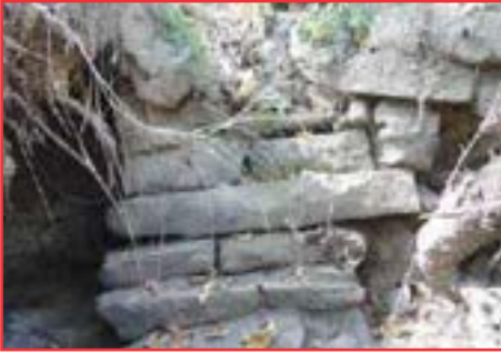
The check dam found in sector 29 of Lohgarh Fort.
