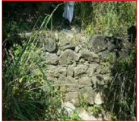
The check dam found in sector 22 of Lohgarh Fort
