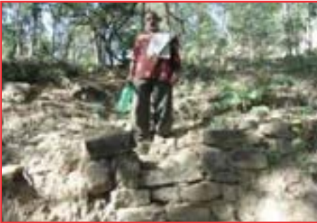
The check dam found in Sector 21 of Lohgarh Fort.
