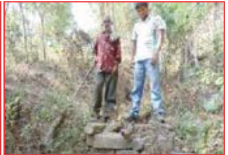
The check dam found in sector 23 of Lohgarh Fort.
