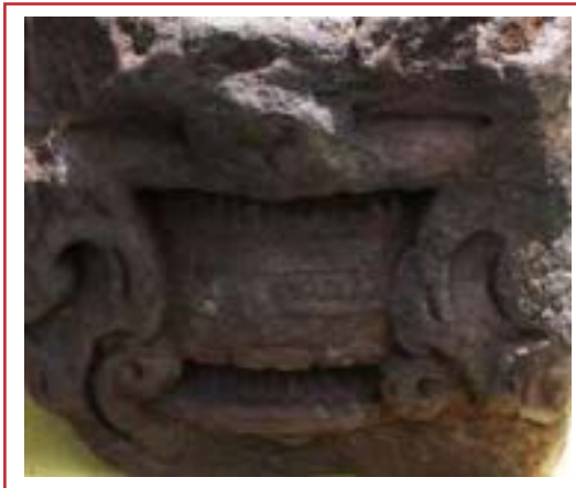
Dressed stone used for construction of fort Lohgarh. There is hole in every stone so that lime mortar can get its strength and each stone are bound with other one strongly.
