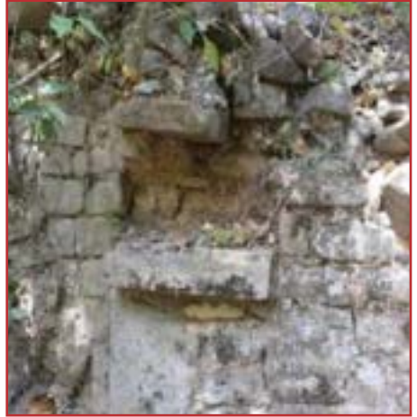
Fort wall having lamp keeper.
