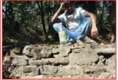
The check dam found in sector 19 of Lohgarh Fort.
