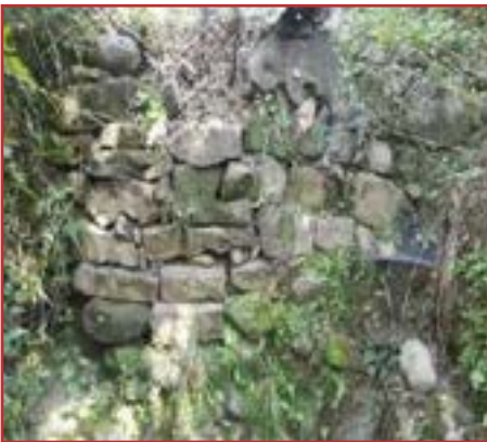
The check dam found in sector 17 of Lohgarh Fort.
