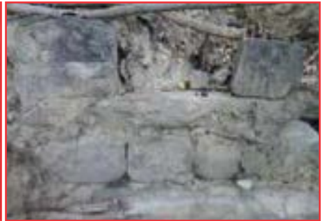
The check dam found in sector 24 of Lohgarh Fort.
