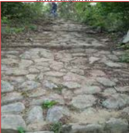
Ramp found in sector C-20
