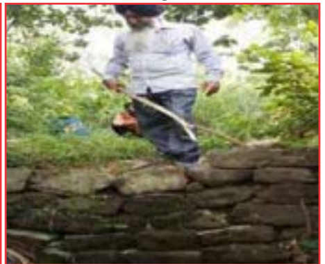
The check dam found in sector 2 of Lohgarh Fort.
