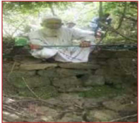
The check dam found in sector 15 of Lohgarh Fort.
