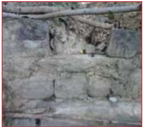
The check dam found in sector 23 of Lohgarh Fort.
