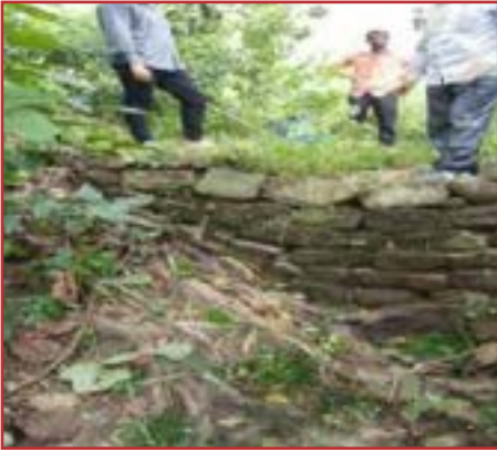
The check dam found in sector 11 of Lohgarh Fort.
